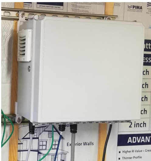
Figure 11. Example Power Enclosure installation on Unistrut across wood studs
