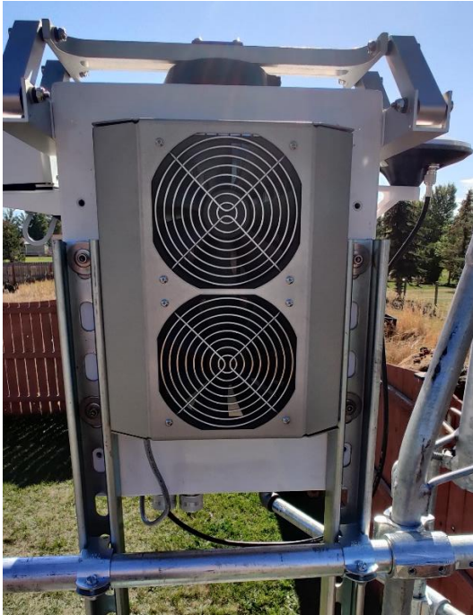
Figure 3. Photo from the back after mounting.
